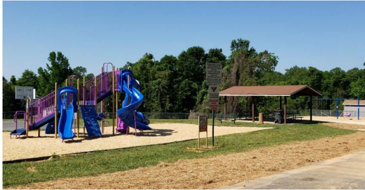
NEW PLAYGROUND EQUIPMENT has been installed at H.K. Griggs Park.
