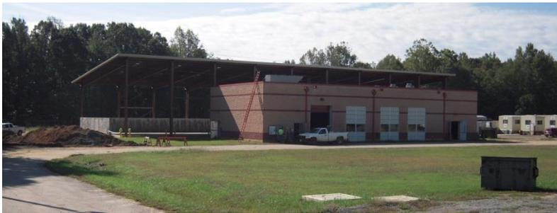
The water and wastewater plant projects continue to proceed with the focus of the work being equipment installation and electrical improvements. The solids handling building is nearly complete on the outside. The primary purpose of the new solids handling building is to house the new drum thickeners and the sludge press, as well as the associated control panels and other electrical gear.
