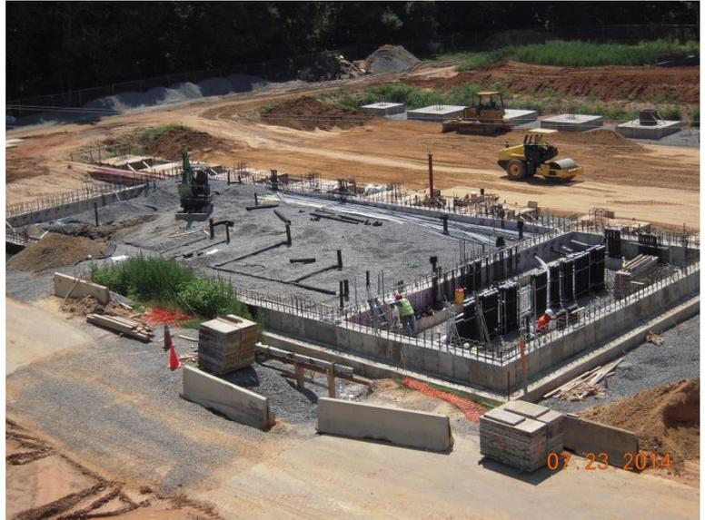
These footings will support a canopy over a separate concrete floor which will be used to store dewatered plant residuals following the dewatering processes. Approximately 6 weeks remain in this portion of the building preparation. Afterwards the walls will begin to go up and we anticipate the building portion to be complete before the end of the year. Once the building is "dried in" then process equipment and electrical equipment installation can start.
